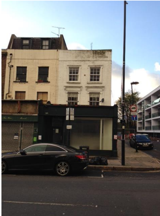
Image 2: View looking west at 325 Caledonian Road
